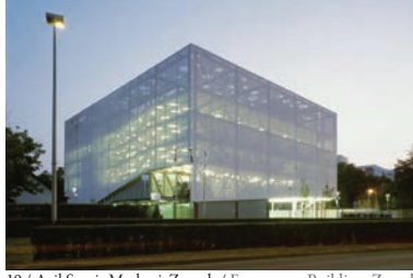
10 / Acil Servis Merkezi, Zagreb / Emergency Building, Zagreb
